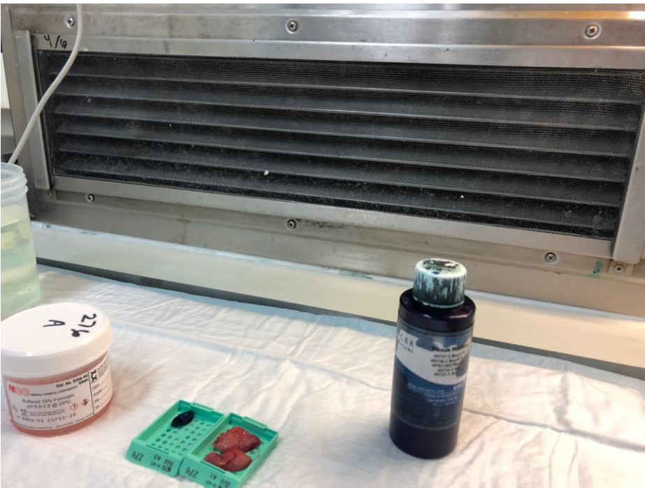
Above: Vents built into wall at grossing stations in LLUMC-Main Campus gross room
